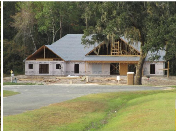
Home under construction in Turkey Ridge – photo James Horton
